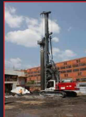
Large Diameter Drilled Shafts
